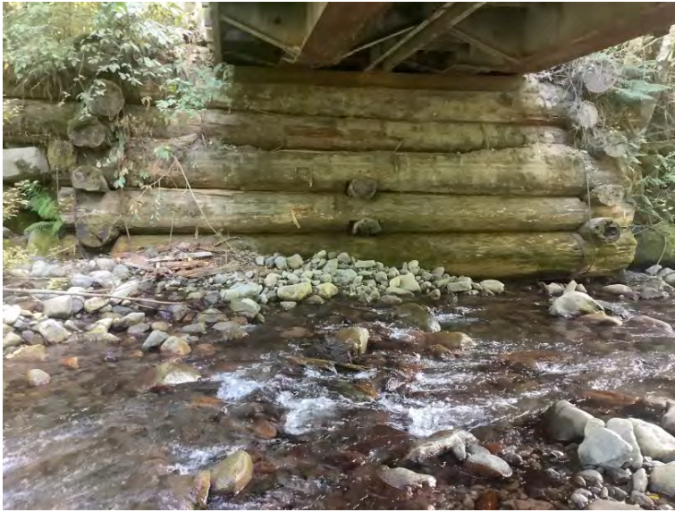
Left Bank Abutment when facing downstream
