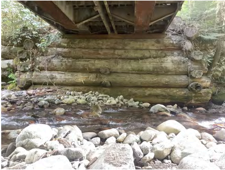
Left Bank Abutment when facing downstream
