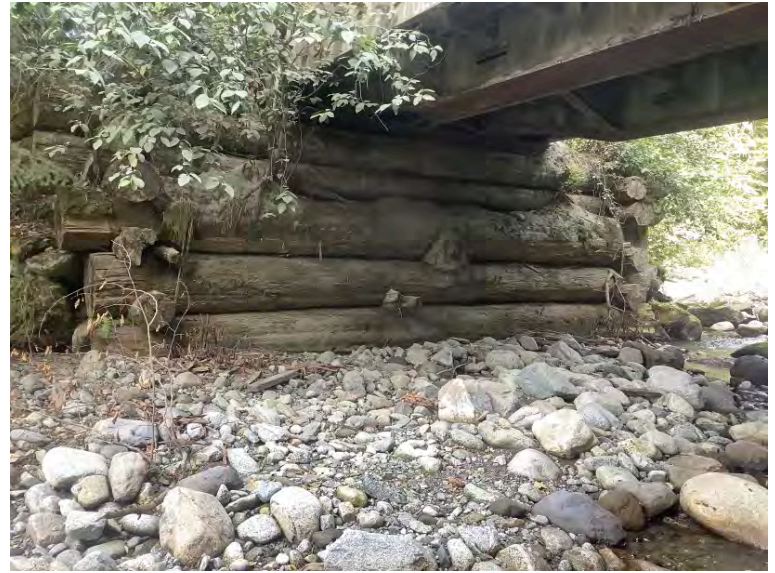
Right Bank Abutment when facing downstream
