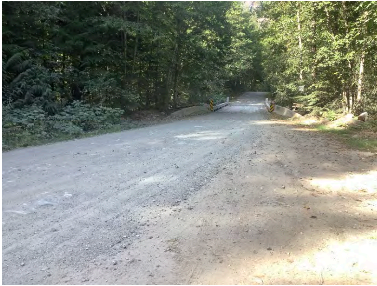
Approach from Left Bank when facing downstream
